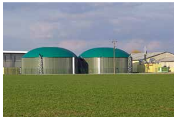
Renewable Natural Gas Plant
